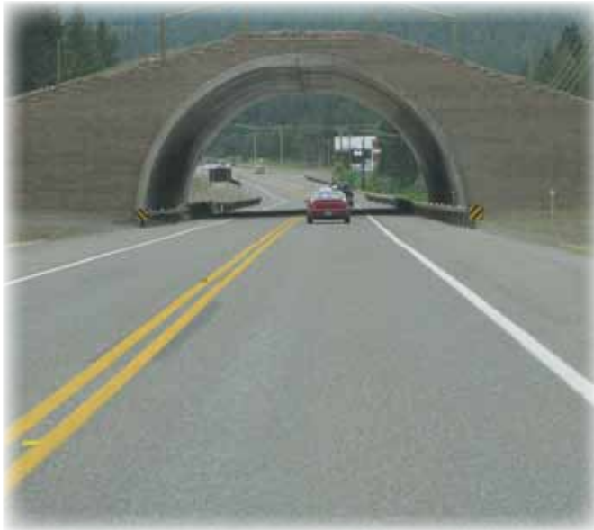
The Peoples Way Overpass
