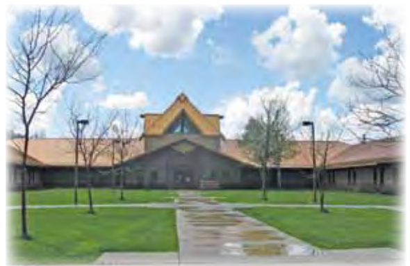
Northern Cheyenne Tribal Administration Building roof improvements
